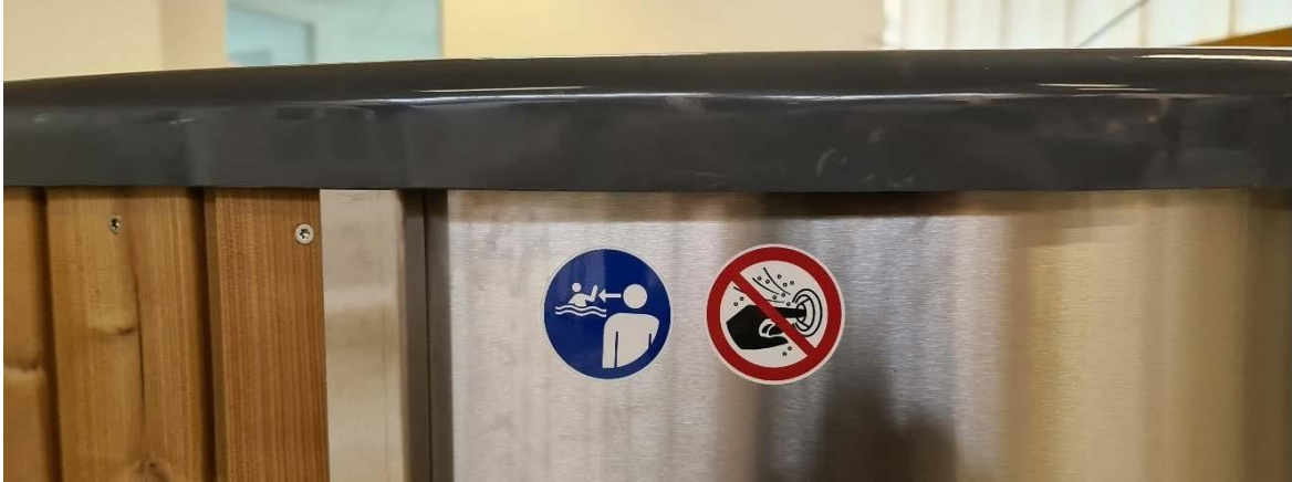
Figure 2: There is no warning attached to the hot tub regarding supervision of children and prohibition of sticking fingers into the jets..
