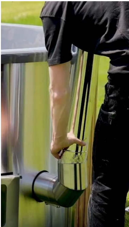
Figure 16: Assembling the lower pipe
