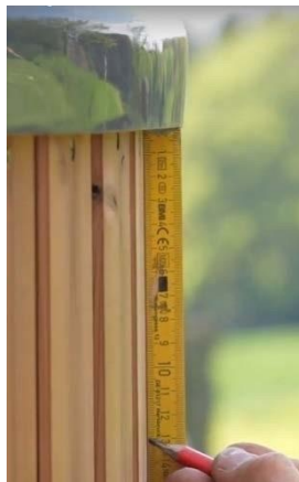
Figure 18: Scope of delivery, marking the assembly position for the top edge of the shelf brackets, positioning of the shelving board
