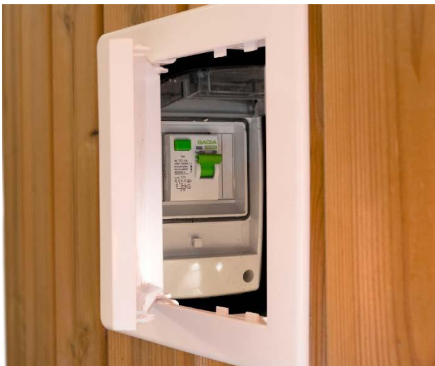
Figure 23: Position and illustration of the RCD (switched on)
