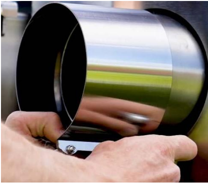
Figure 15: Fastening the fixing clamp to the stove spigot
